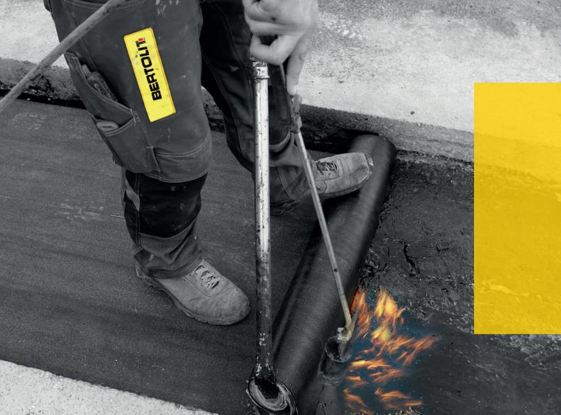
**L'ÉTANCHÉITÉ DES TOITURES, DES TERRASSES, BALCONS ET PARKINGS DOIT ÊTRE FIABLE POUR ÉVITER D'IMPORTANTES DÉGRADATIONS DES BÉTONS CONNEXES**
